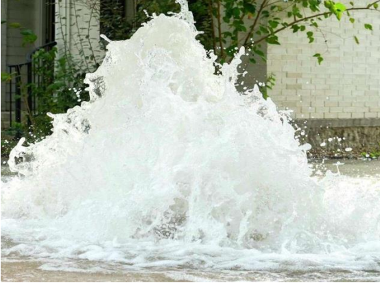
Drought Water Leaks
